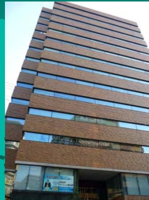
HQ's office in Osaka
