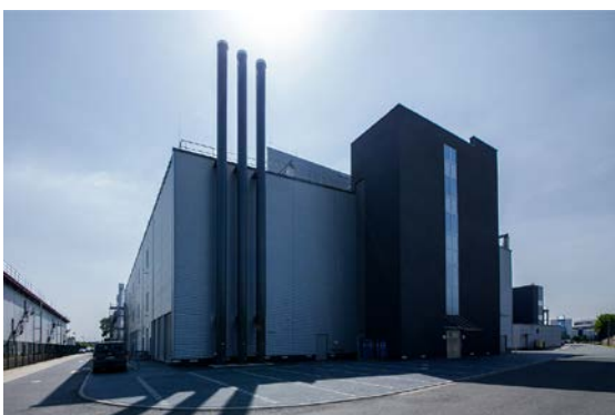
Datacenter Campus in Frankfurt
