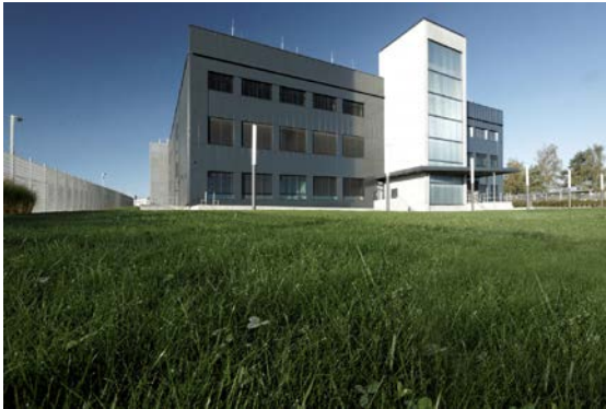
Datacenter in Zurich
