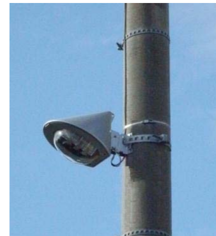
(施工例) LED防犯灯
