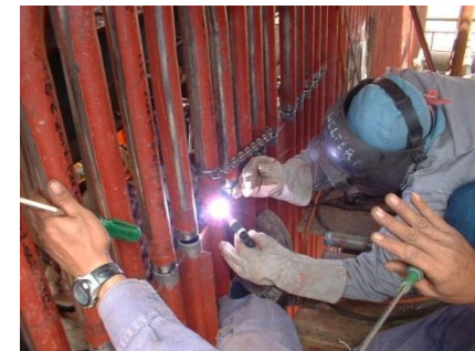
溶接施工一例
