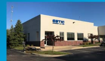
Novi Technical Center
