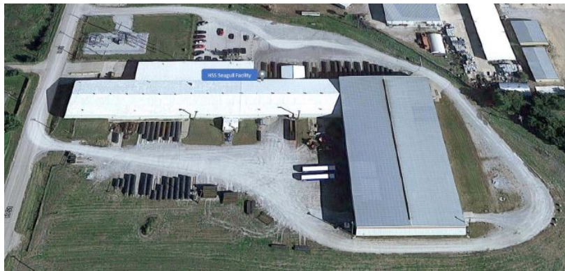
Geneva Structural Tubes,LLC (GENEVA社)
