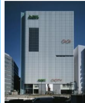
Shinjuku 3-Chome East Building
