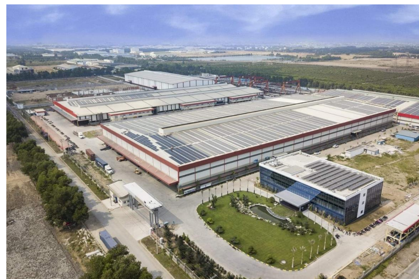
Dai Dung An Ha Factory roof top (Thang Long Power)/Vietnam
