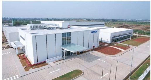
工事名：Design & Construction of Healthcare Manufacturing Facility – Project Horizon(インド) 施主名：OMRON HEALTHCARE MANUFACTURING INDIA PRIVATE LIMITED(オムロンヘルスケア株式会社)
